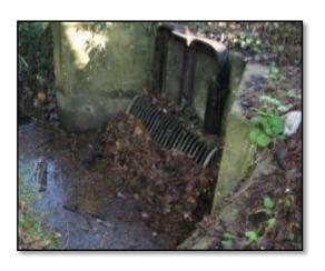
• Culvert entrances and exits often have protective grilles to prevent debris entering the pipe and causing blockages. These should be inspected and cleared regularly, especially during the winter or periods of heavy rainfall when debris can accumulate very quickly.
